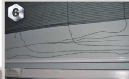
**6** My problem was that the top two cords were broken near to the fixed edge of the door (See diagram at point X). These two cords are in fact one cord that forms a loop and joins a third cord (the bottom drawstring) in the leading edge
