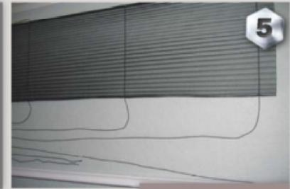
**5** The black concertina screen itself is held in position by being slid into a groove in the leading edge door extrusion (the bit you slide to open or close the door). And the other side of the screen is held in position in the same manner in the fixed edge, which does not move
